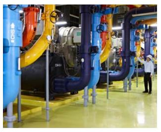
With closed cell structure, low thermal conductivity, low water absorption and flame resistance. Aeroflex is widely used in chilled water cooling system in high standard buildings.
