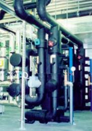
Because of low water absorption and water vapor transmission, Aeroflex is widely used in heating and cooling system.
