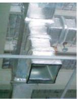
Aeroflex can work efficiently as an sound dampening material when used as internal and external insulation for medium and high velocity air duct system.
