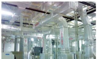
Neat appearance when used as external insulation for air ducts in phamasutiocal laboratory facility.
