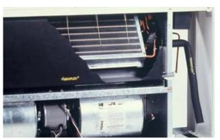
Aeroflex does not contain any fibrous material, so it is safe to use in direct contact with air, provides the excellent IAQ (Indoor Air Quality) Standard.
