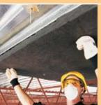
Wall and Ceiling Liner M is commonly used to provide an acoustical treatment in theaters and concourses. It is also used as a ceiling cover in small restaurants for visual aesthetics.
